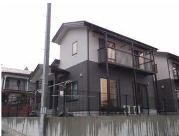
■岩手縣大槌町吉里吉里A公營住宅2017年6月完工 The A public housing units in Kirikiri, Otsuchi, Iwate Prefecture were completed in June 2017
