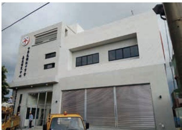
■新落成的嘉義備災中心 The newly completed Chiayi Disaster Preparedness Center
