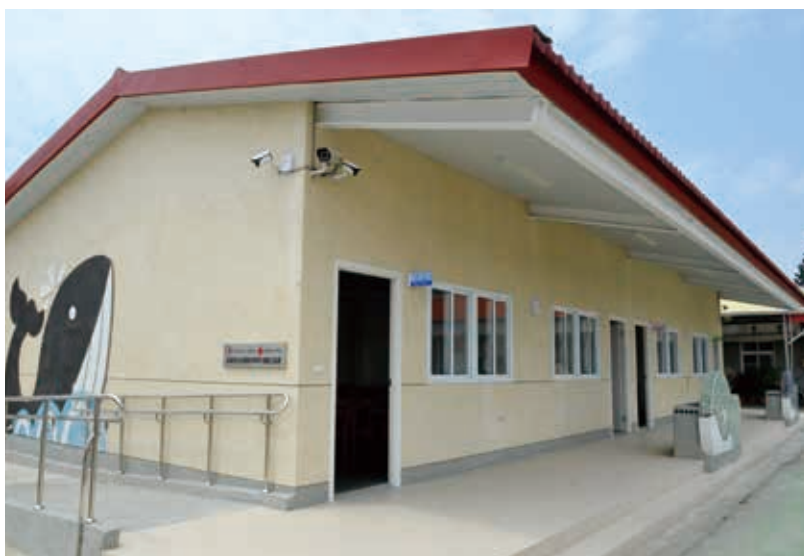
■臺南市北門國小西棟教室完成重建 Reconstructed western classroom building at Bei-Men Elementary, Tainan City
