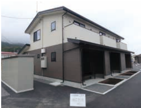
■岩手縣大槌町浪板魚集公營住宅2017年8月完工 The Fishery Dist. public housing units in Namiita, Otsuchi, Iwate Prefecture were completed in August 2017
