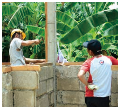
■ 重建房屋，巴蓋村民一起來 Rebuilding homes together with the villagers of Bagay
