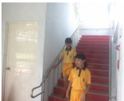
■教學樓左側樓梯重建後寬敞安全 The stairs on the left side of the classroom building are spacious and safe after reconstruction
