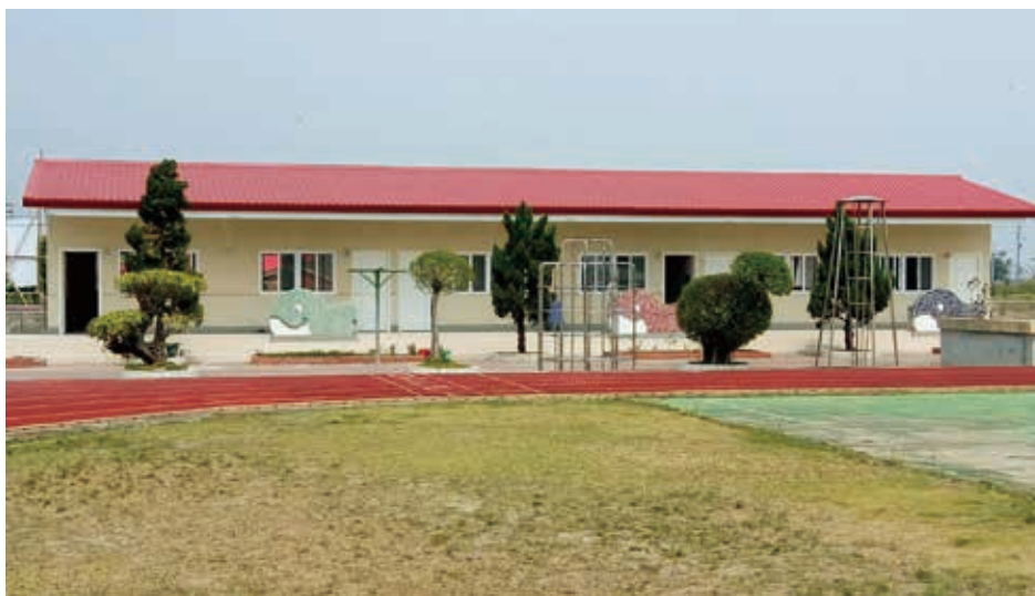
■臺南市北門國小玉湖分校北棟教室完成重建 Reconstructed northern classroom building at Bei-Men Elementary's Yu-Hu Campus, Tainan City
