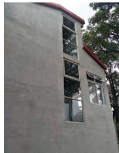
■教學樓原本殘破不堪，整修後牆面全新 Originally destroyed, the walls of the classroom building are now completely new
