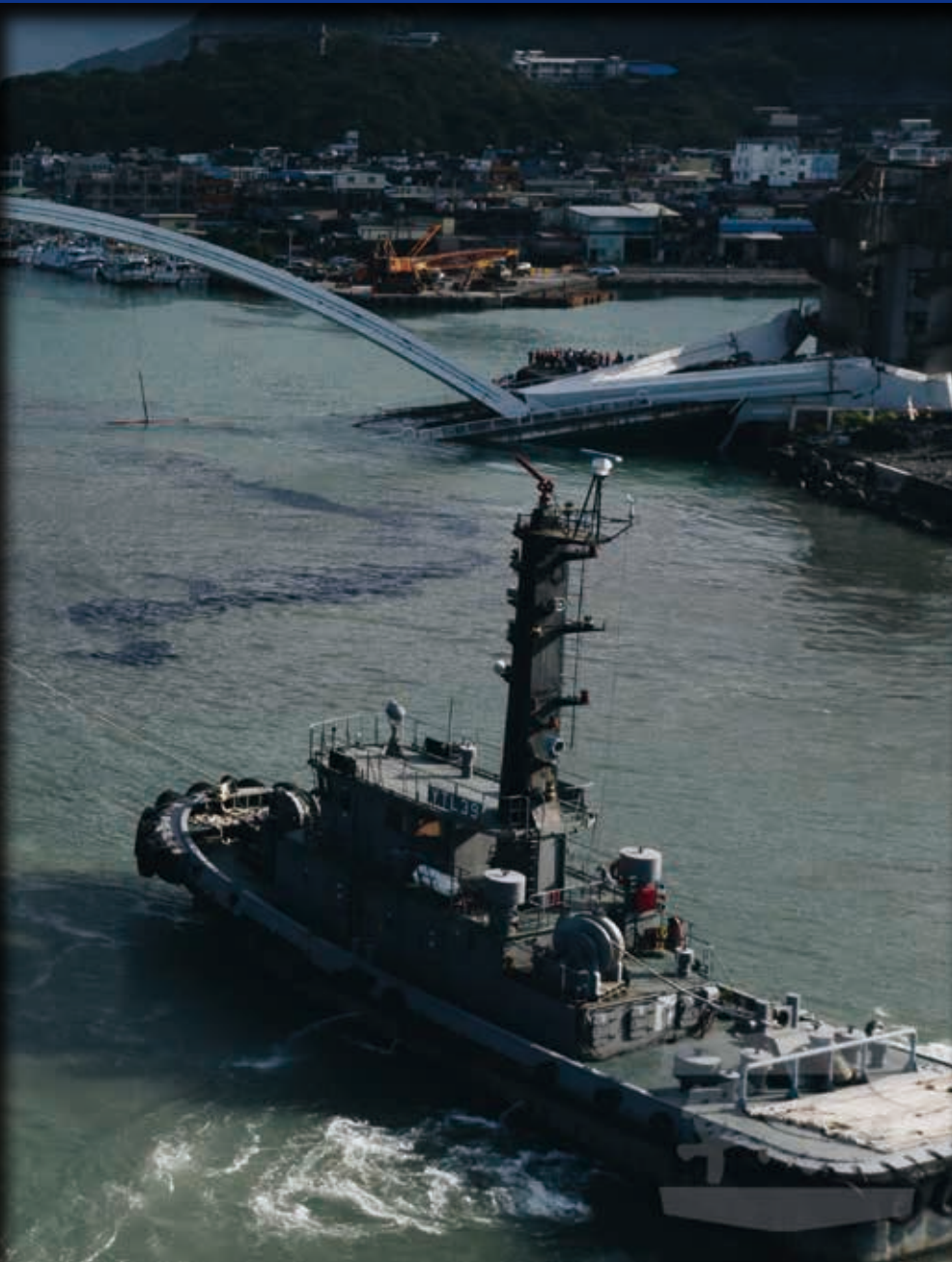
斷橋事件發生後，軍方於宜蘭南方澳大橋進行救援任務(軍聞社提供) Military conducts search and rescue operations after the Nanfang'ao Bridge in Yilan County collapsed (Photo credit: Military News Agency)
