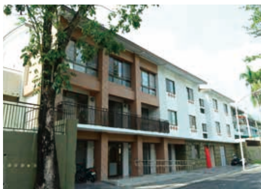
高雄市甲仙國中教職員宿舍造價約3,669萬元，1樓有交誼廳、廚房和小型備災倉庫 Jia-Sian Jr. High's faculty dormitory cost NTD 36 million to build, boasts a common room, kitchen, and compact disaster preparedness warehouse
