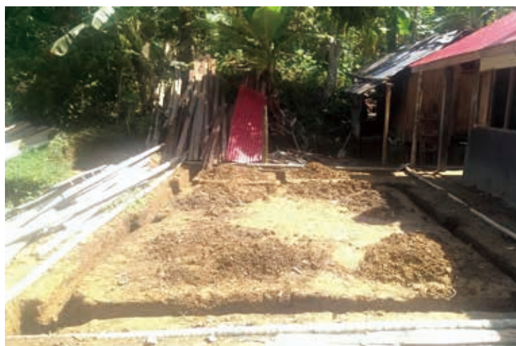
正進行排水管線施工的核心住宅 One of the houses undergoing plumbing installation
