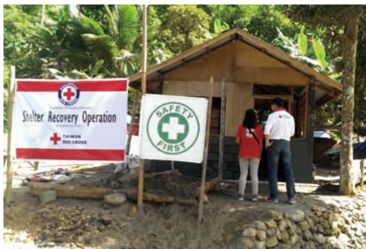
援建的核心住宅只差粉刷外牆即可完工 The housing is almost complete, only lacking a coat of paint on its exterior
