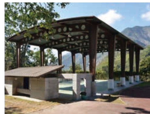
樟山國小風雨球場為開放式鋼構設計，天災來臨時可配合堆放賑濟物資 Changshan Elementary's covered ball court was designed so that it can be used as a gathering site for relief supplies during disasters
