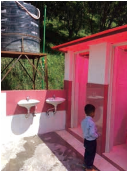
本會為加德滿都孤兒院迅速興建完成4間廁所 We assisted in the construction of 4 latrines at an orphanage in Kathmandu
