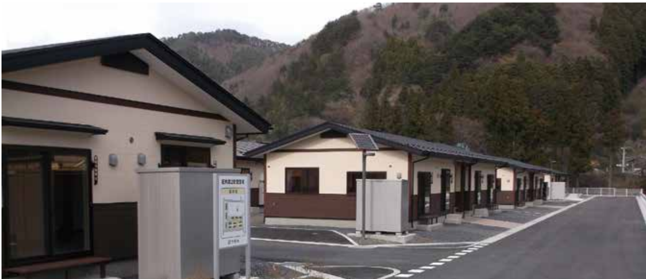
■岩手縣大槌町柵內第2公營住宅2016.3完工 The No.2 public housing units in Masanai, Otsuchi, Iwate Prefecture was completed in March 2016.
