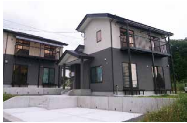
■岩手縣大槌町波板第1公營住宅2016.6完工 The No.1 public housing units in Namiita, Otsuchi, Iwate Prefecture was completed in June 2016.
