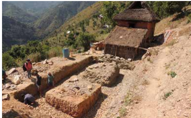
■耐久屋正在進行挖基底置放地樑工程 Construction of durable shelters: topping foundations with ground beams.
