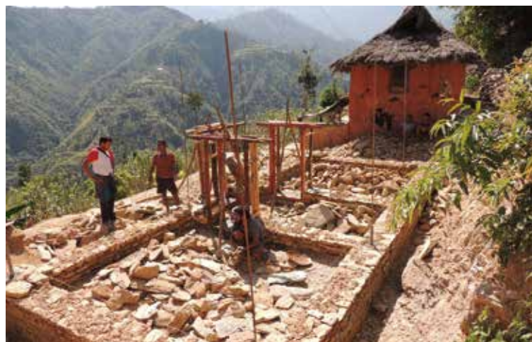
■耐久屋地樑砌石打地坪大功告成 Floor level stone masonry construction has been completed.
