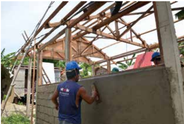
■ 北宿霧巴蓋村核心住宅施工狀況 The construction of core shelters in northern Cebu.
