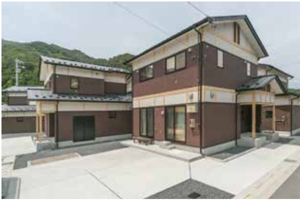
■岩手縣大槌町寺野第2公營住宅2016.6完工 The No.2 public housing units in Terano, Otsuchi, Iwate Prefecture was completed in June 2016.
